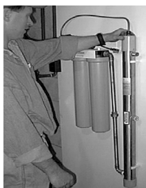
Install UV unit
